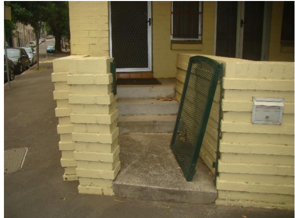
Plate 4. Elevated access at NE corner of northern lot.
