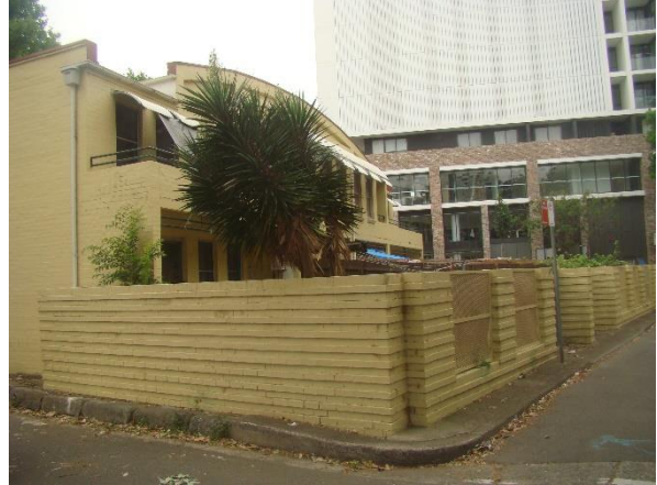
Plate 2. Structure occupying northern lot with central lane.
