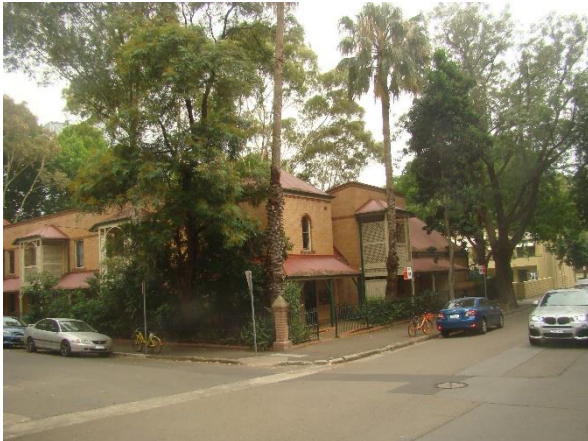
Plate 7. Structure occupying southern lot.
