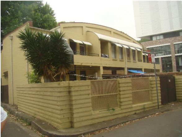
Plate 3. Structure occupying northern lot.
